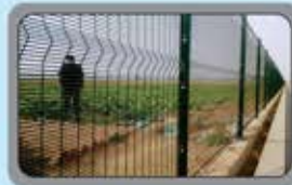
Anti Climb Fence
