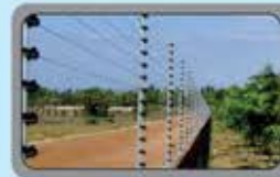
Weld mesh Fencing
